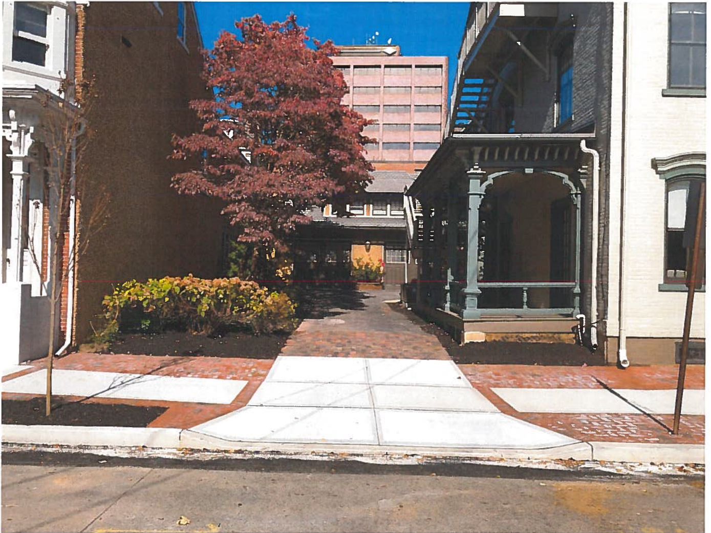
Existing access drive on the property. The project includes the reinstallation of an existing gate at this entrance.
